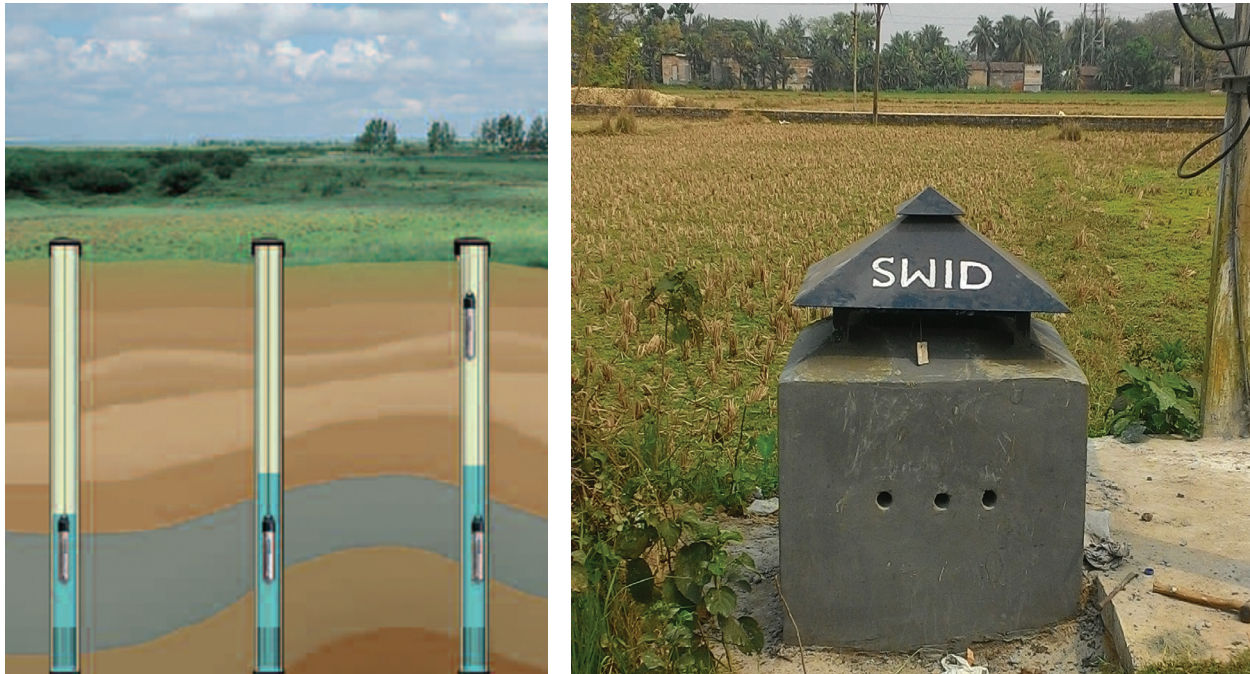
Figure 4.1: a) Water level installed in multiple aquifers; b) the secured structure for telemetry designed by the State Water Investigation Directorate, Government of West Bengal (right)
